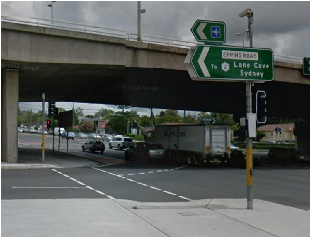
Figure 37 Lane Cove Road / Epping Road overpass
