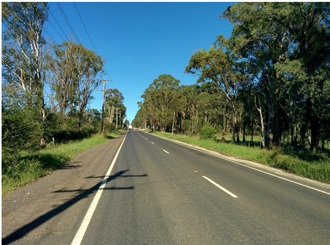
Figure 7 Garfield Road East
